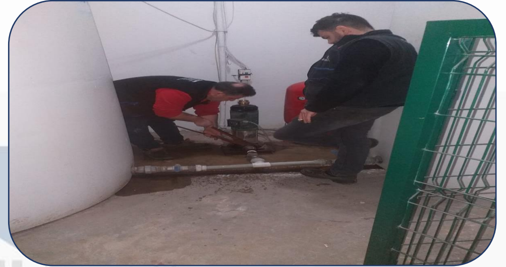
The Renewed Expansion Tank In Block A
