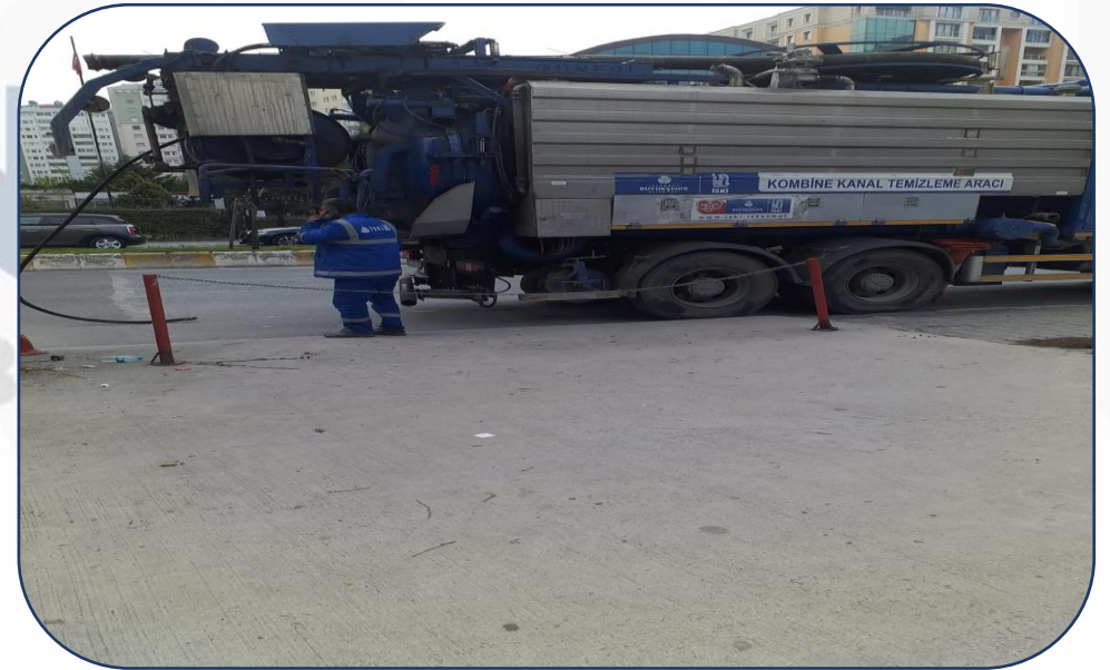
Cleaning Of Wastewater Drains
