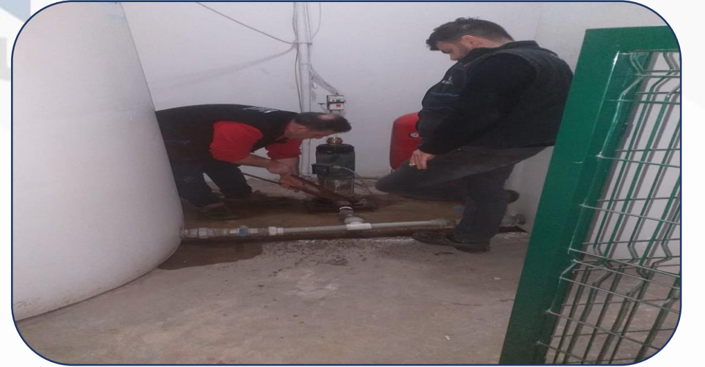
Replacing the Check Valve
