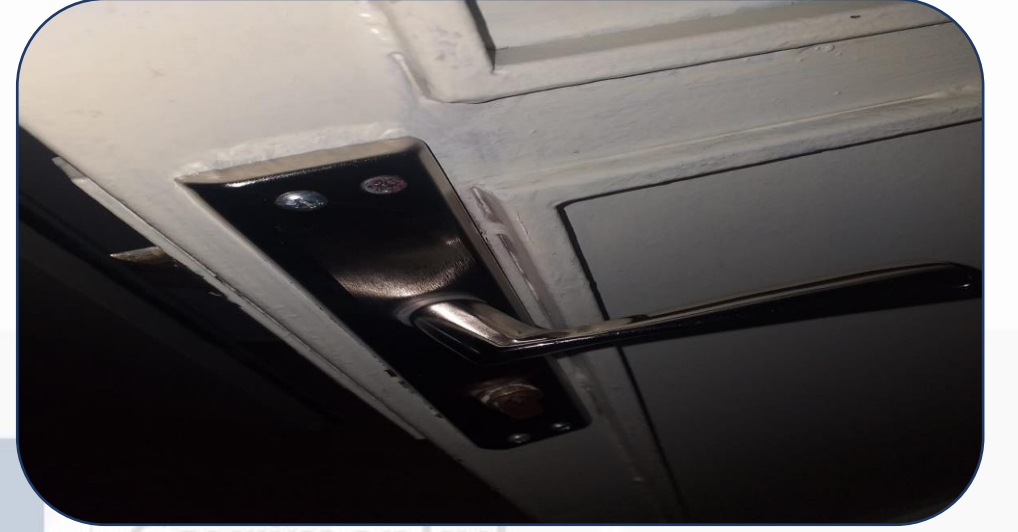
Replacement of Door Handle
